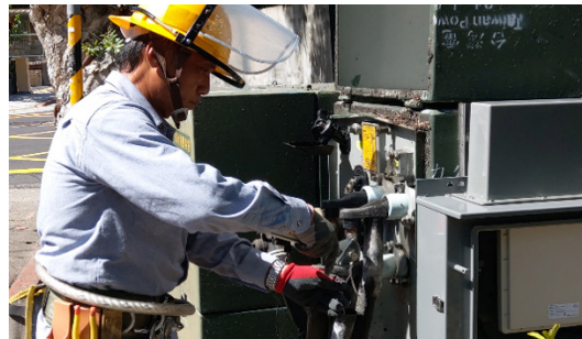
Figure 6: On the top, meter and communication module installation. On the bottom, ground level base station installation.
