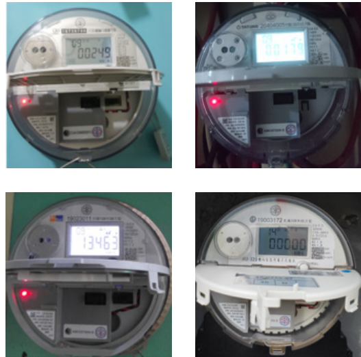
Figure 2: Examples of some existing meters into which Ubiik's technology has been integrated.
