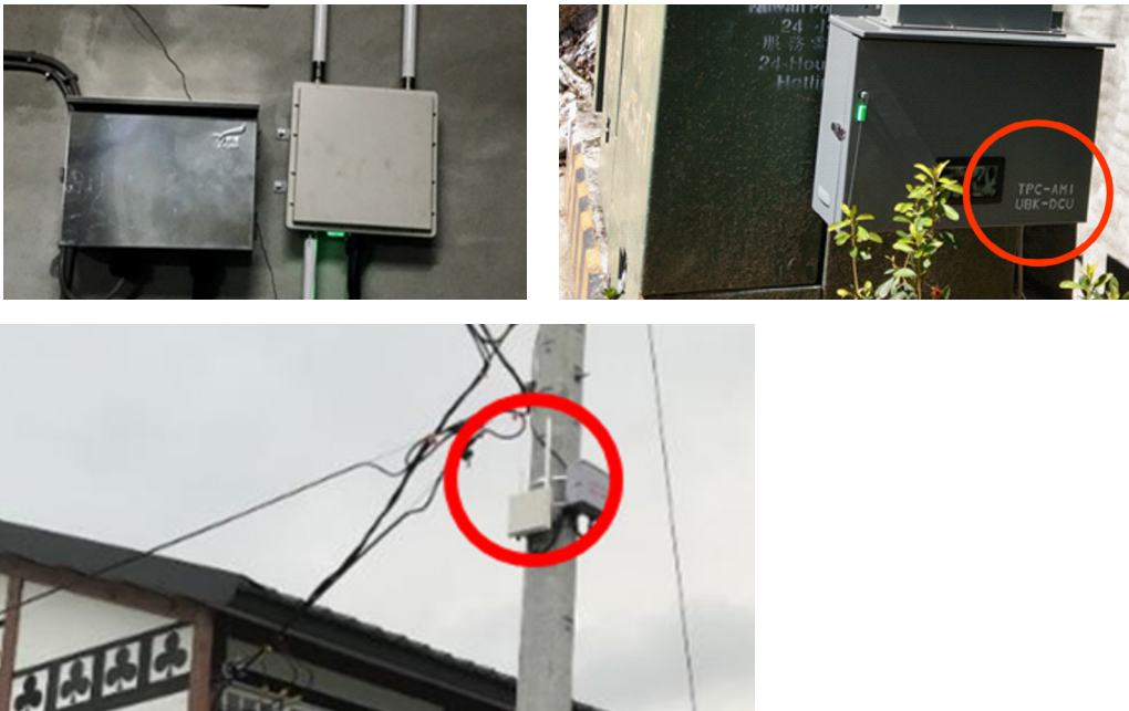
Figure 5: DCUs installed at three different locations in Taiwan. Ubiik provides 320 DCUs to provide communication that will provide service to roughly 280,000 FAN devices in Taiwan by the end of 2020. Middle location is a pole mounted DCU, while right location is mounted at ground level.
